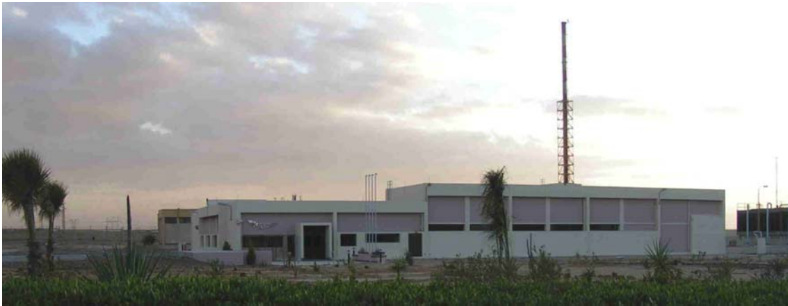
Fig. 10 – Radioisotope Production Facility (RPF) inside Inshas Atomic Center - Egypt
