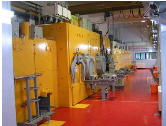
Fig. 12 – View of the hot corridor -RPF Egypt
