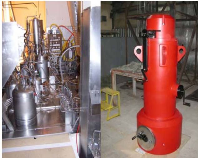
Fig. 17 – New process equipment and Filter Transfer Flask –ANSTO Moly
